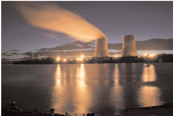
Watts Bar Nuclear Plant
