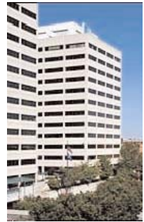
The OIG is primarily located in the TVA Towers in Knoxville.
