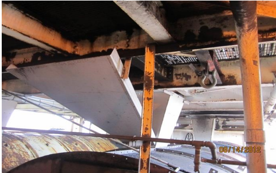
Picture 2: A spill pan as observed at CUF on August 14, 2012, in the Rotary Breaker building. Spill pans help eliminate accumulation of coal dust.
