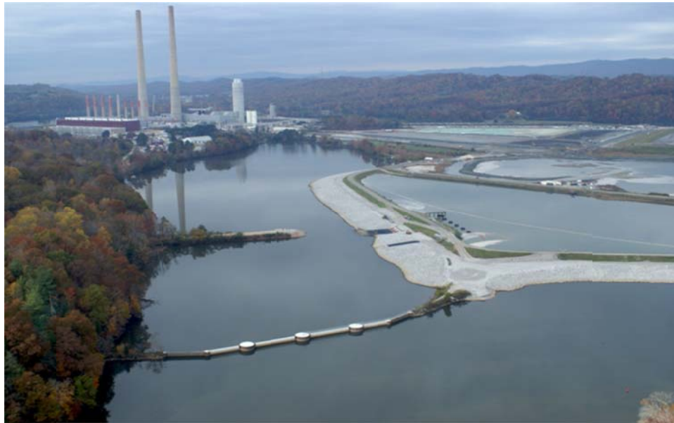
Figure 4: Skimmer Wall and Intake Channel
