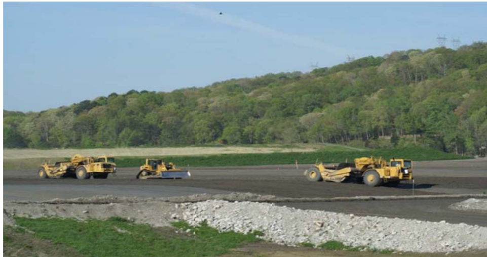
Figure 6: Ash Stacking in On-site Disposal Area
