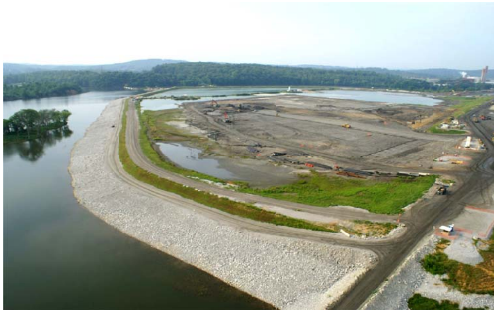
Figure 2: Completed Dike C
