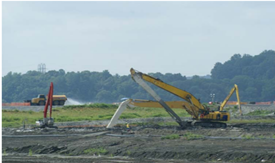
Figure 5: Construction of the PWS
