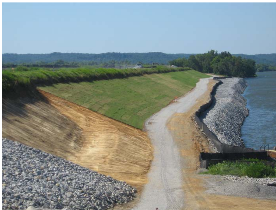
Photo 2 Northeast Dike just prior to completion.
