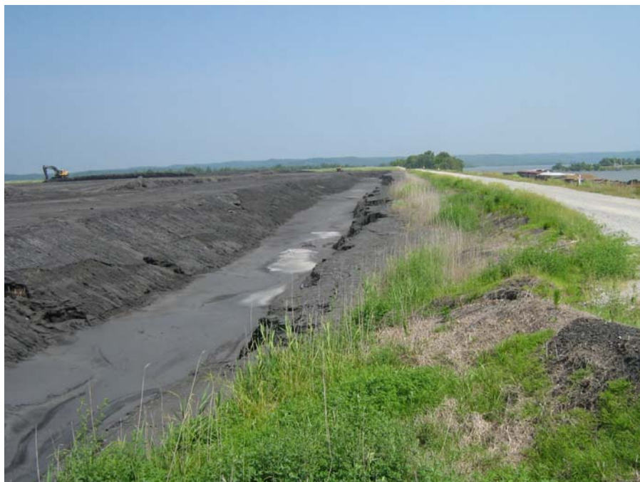
Photo 10 Former sluice channel now dewatered and unused along the Northeast Dike (viewed looking north).
