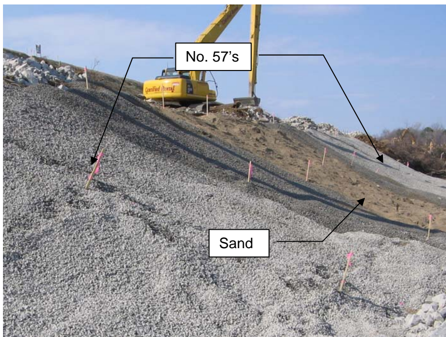
Photo 7 Filter layers placed during construction.
