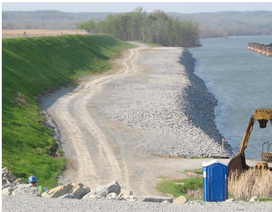
Photo 5 Riprap buttress after completion and prior to dike regrading.
