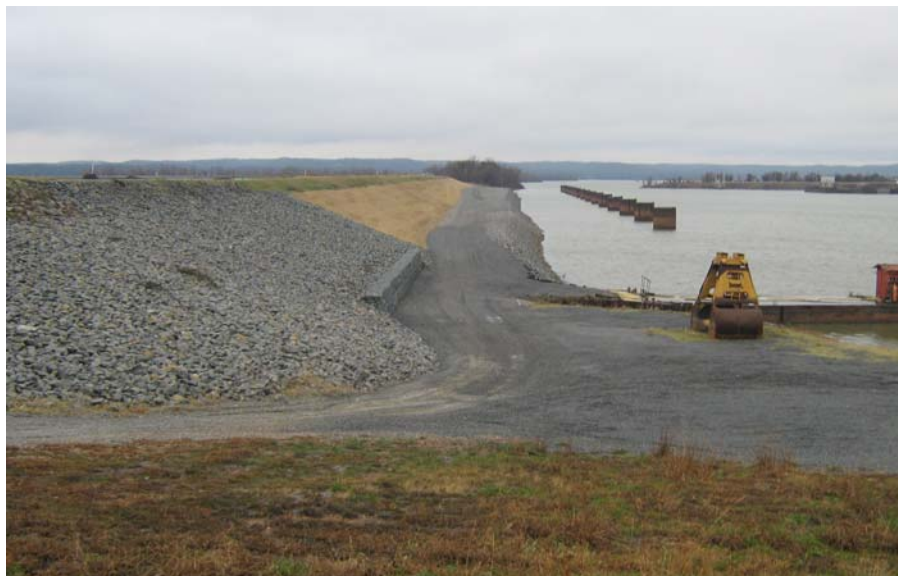
Photo 1 Northeast Dike after improvements.
