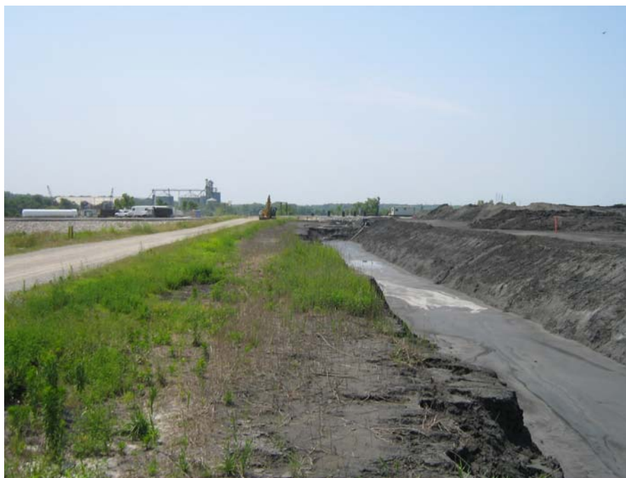
Photo 9 Former sluice channel now dewatered and unused along the Northeast Dike (viewed looking south).
