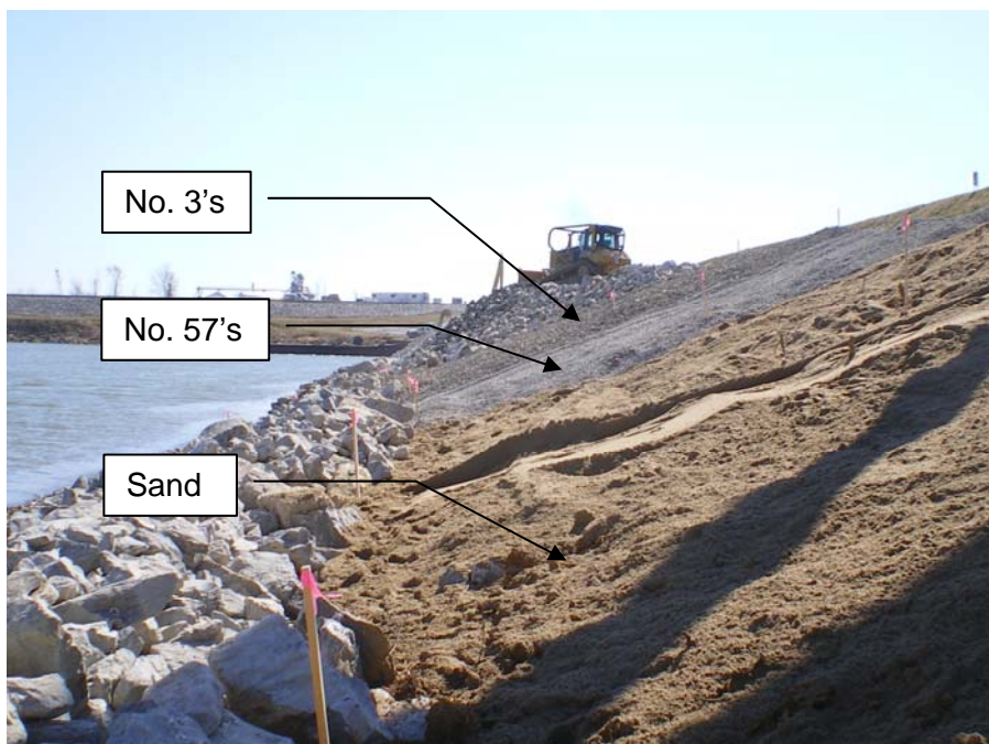
Photo 6 Filter layers being placed during construction.
