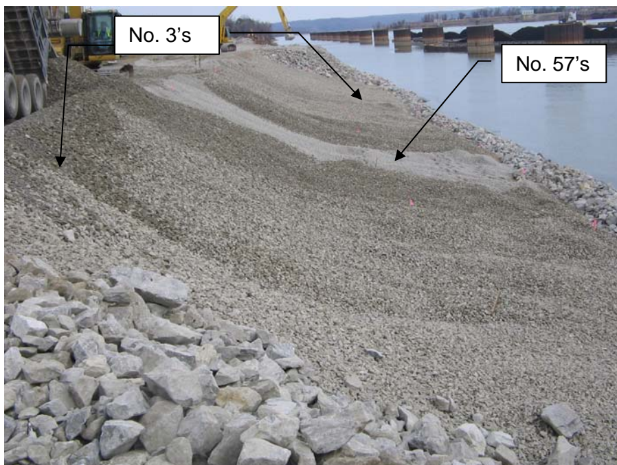
Photo 8 No. 3 stone filter layer being placed over the No. 57 stone layer.
