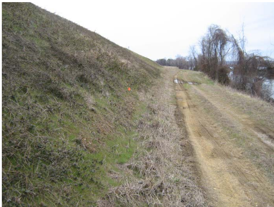
Photo 3 Northeast Dike prior to remedial construction.
